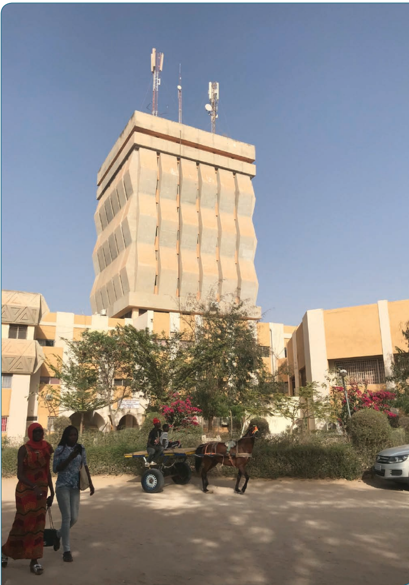
WaziGate deployment on top of UGB tower
